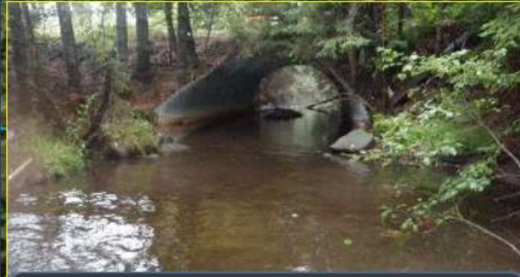
Undersized Culvert = Downstream erosion/sediment transport issues
