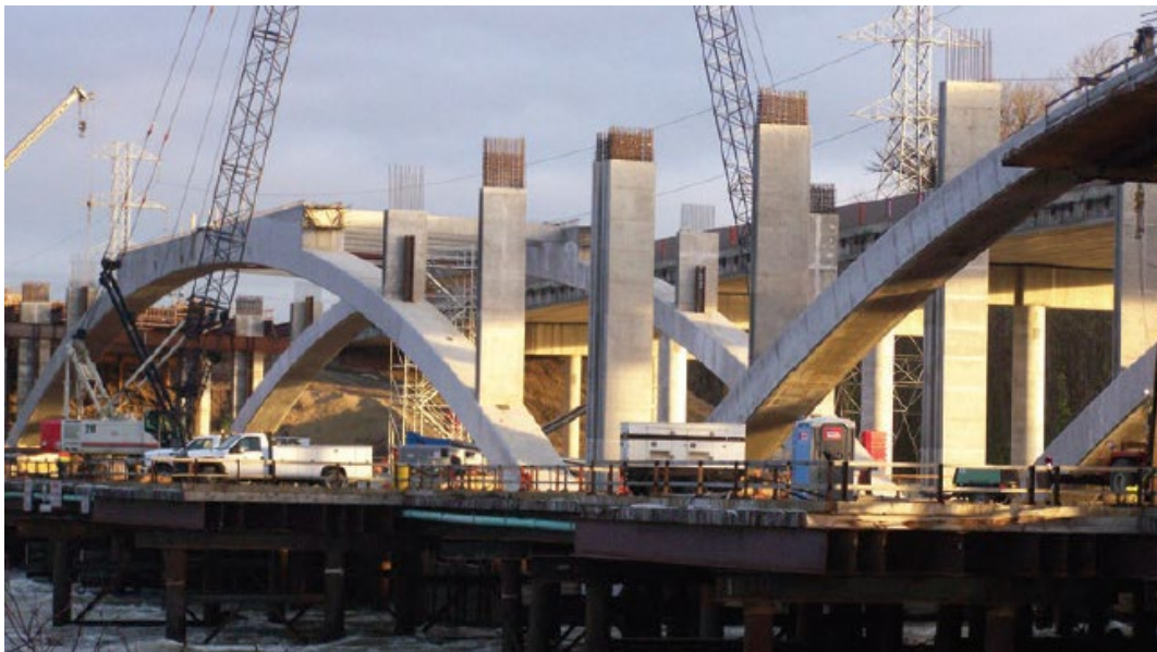
Figure 41. The completed arches of the southbound Willamette Bridge.
