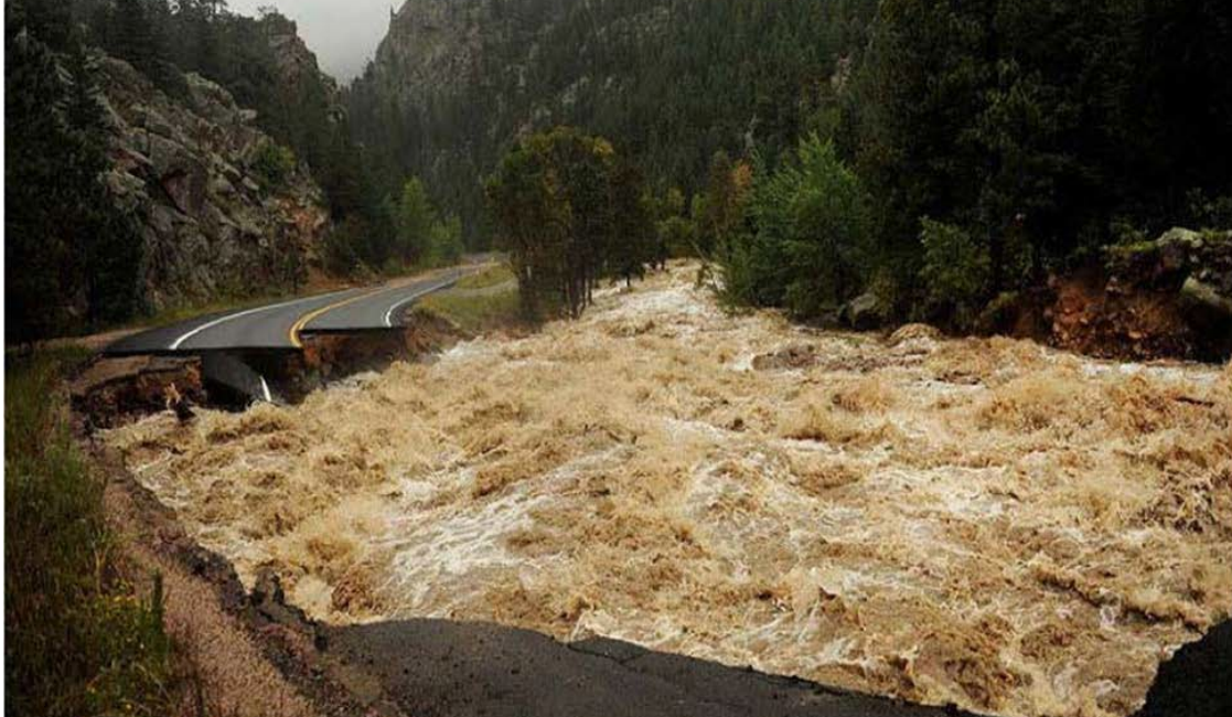
Figure 34. Larimer County Road 43 during flooding. Source: Colorado DOT
