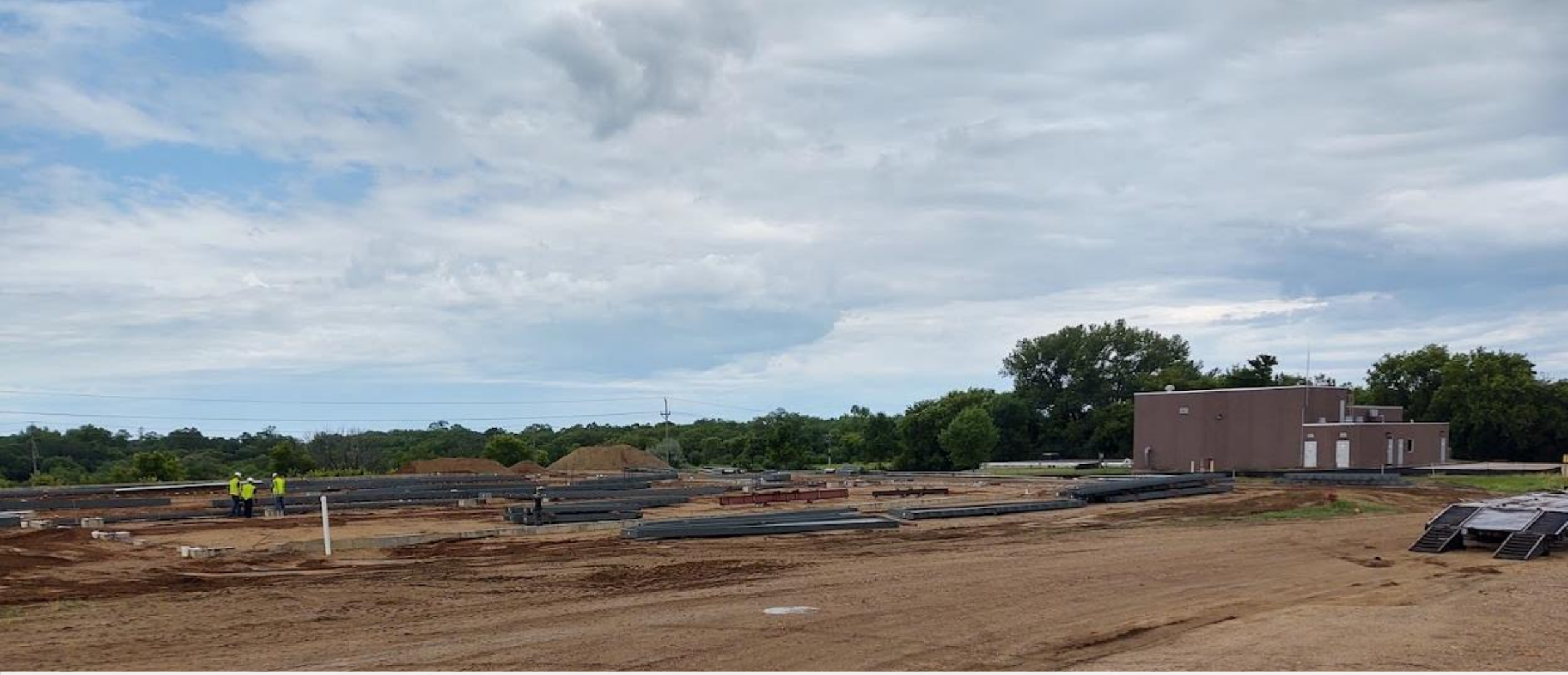
Steel Frame Laid Out
