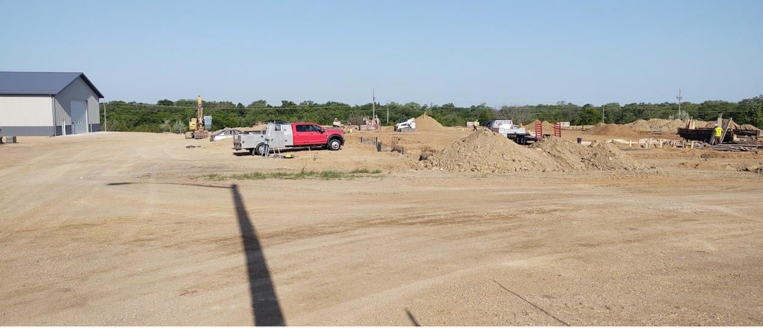
Big Stone Site, footings
