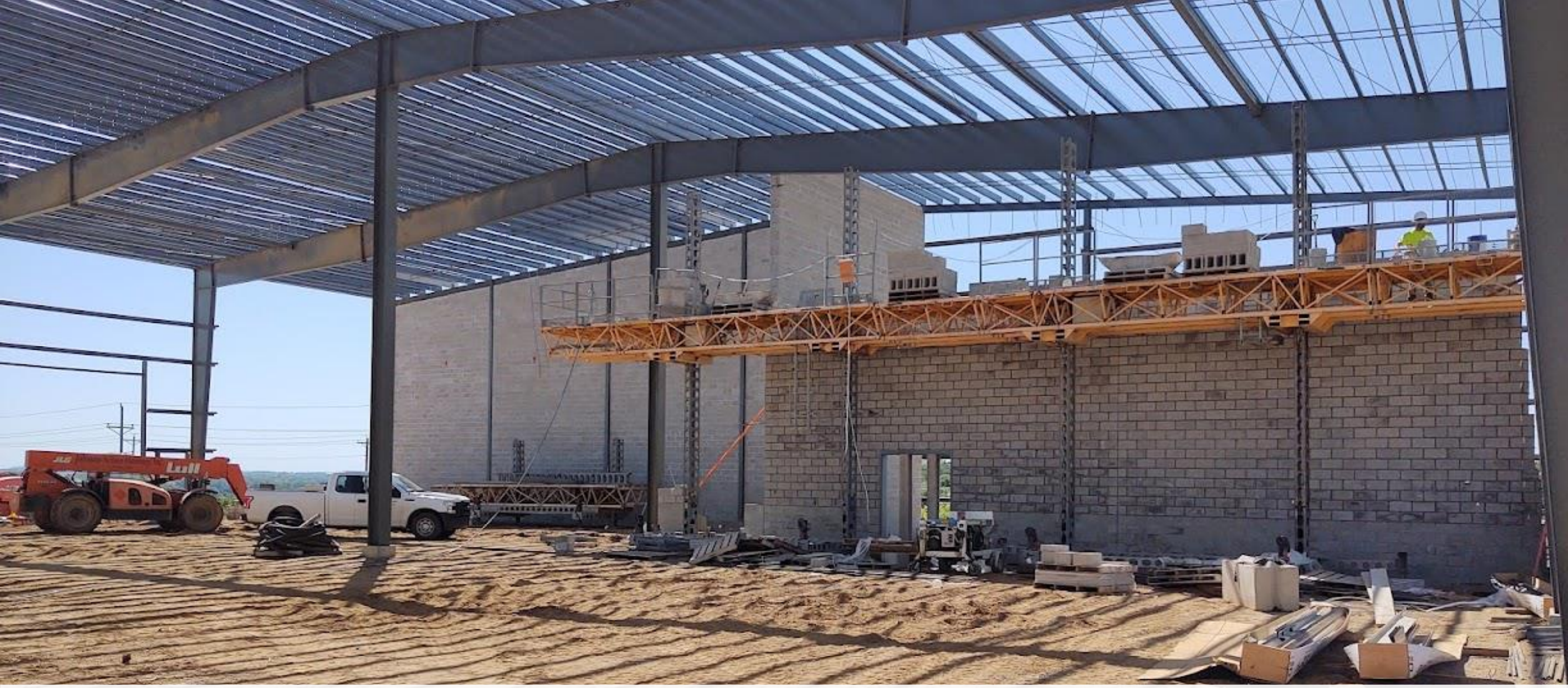
Concrete Masonry Walls going up
