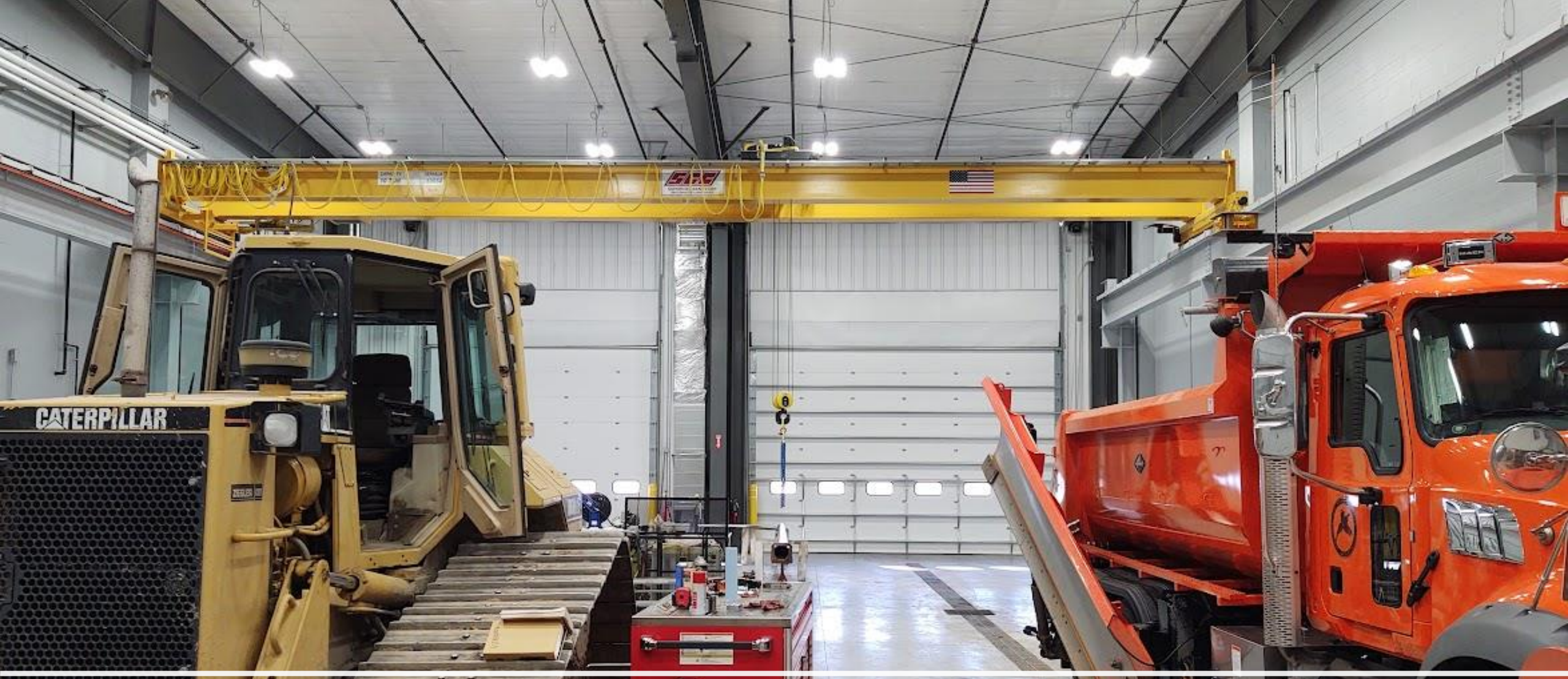
Completed Shop- Big Stone
