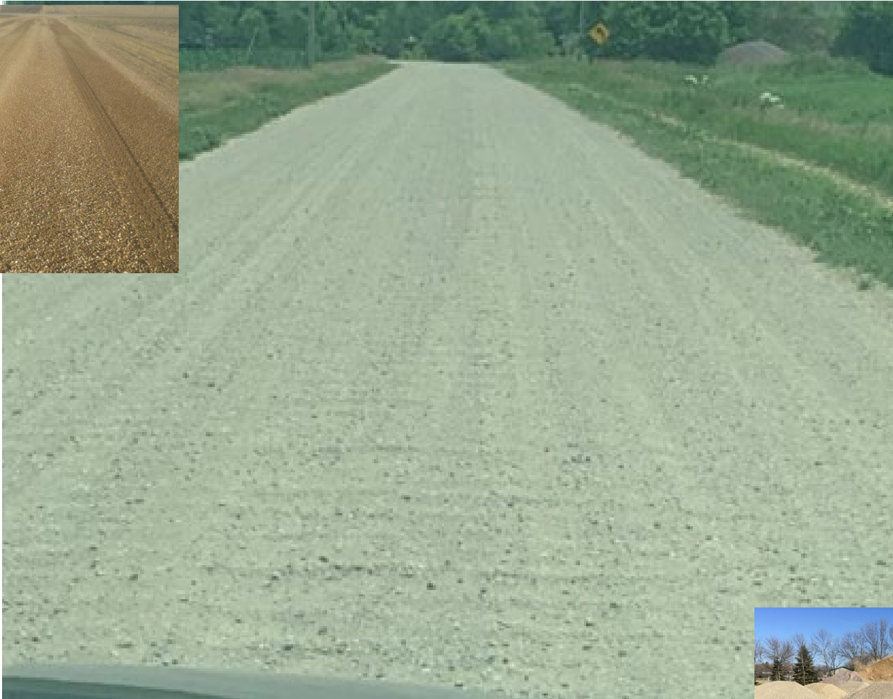
Excessive Loose Surface Rock
