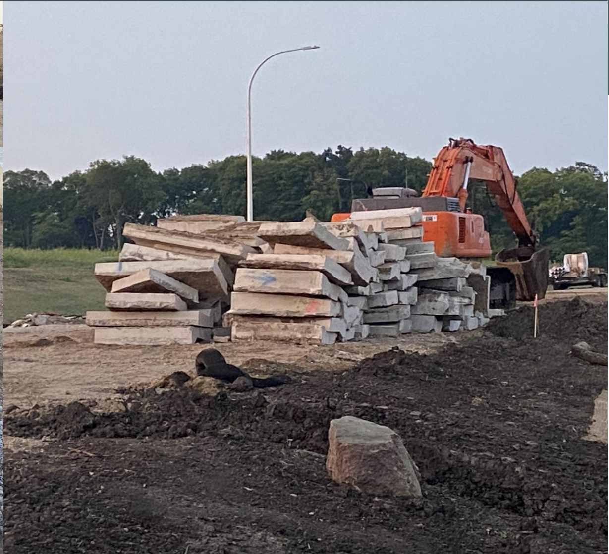
Replacing New Curb & Gutter
